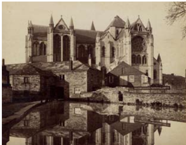
This photograph shows the partly constructed Cathedral in 1887 without its familiar towers and spires. Extensive fundraising was underway to create them, as it is today to restore them!
